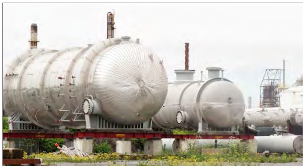
FIGURE 6 Suncor Montreal Coker Equipment in Montreal East.
